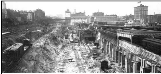
“...The purchases of land made, abutting Lexington, Park and Madison avenues, increased the area from twenty-three acres in the old terminal to seventy-nine acres in the new, including both levels of tracks. As each new track or group of tracks was finished a corresponding number of old ones was abandoned, and traffic went on without interruption...” Scientific American Supplement, December 7 th 1912 13
